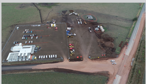
▲ Mortlake South Wind Farm, VIC (under construction)
